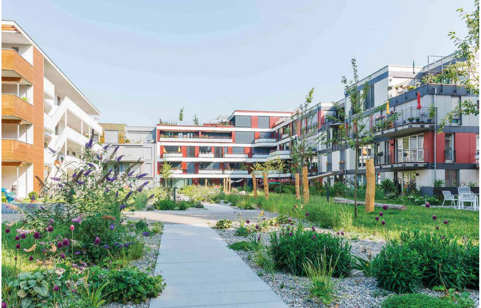
View of courtyard no. 1 with the "Cambium", "Licht und Luft", "Neckarblick" and "Open" projects. Architecture: bsarchitektur, Wamsler Architekten, Baisch+Fritz Freie Architekten, Krisch Partner. Photo: Peter Jammerneegg
