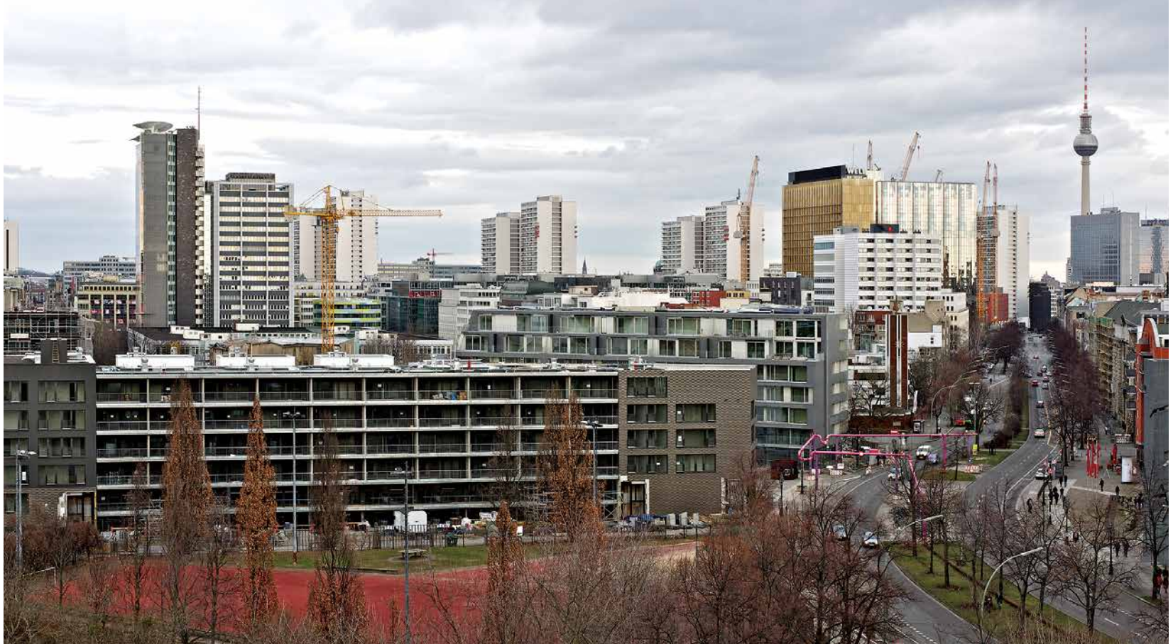
Integrated building project on the site of the former wholesale flower market (IBeB). Architects: Arge ifau (Institut für angewandte Urbanistik) and HEIDE & VON BECKERATH; client: IBeB GbR. Photo: Andrew Alberts
