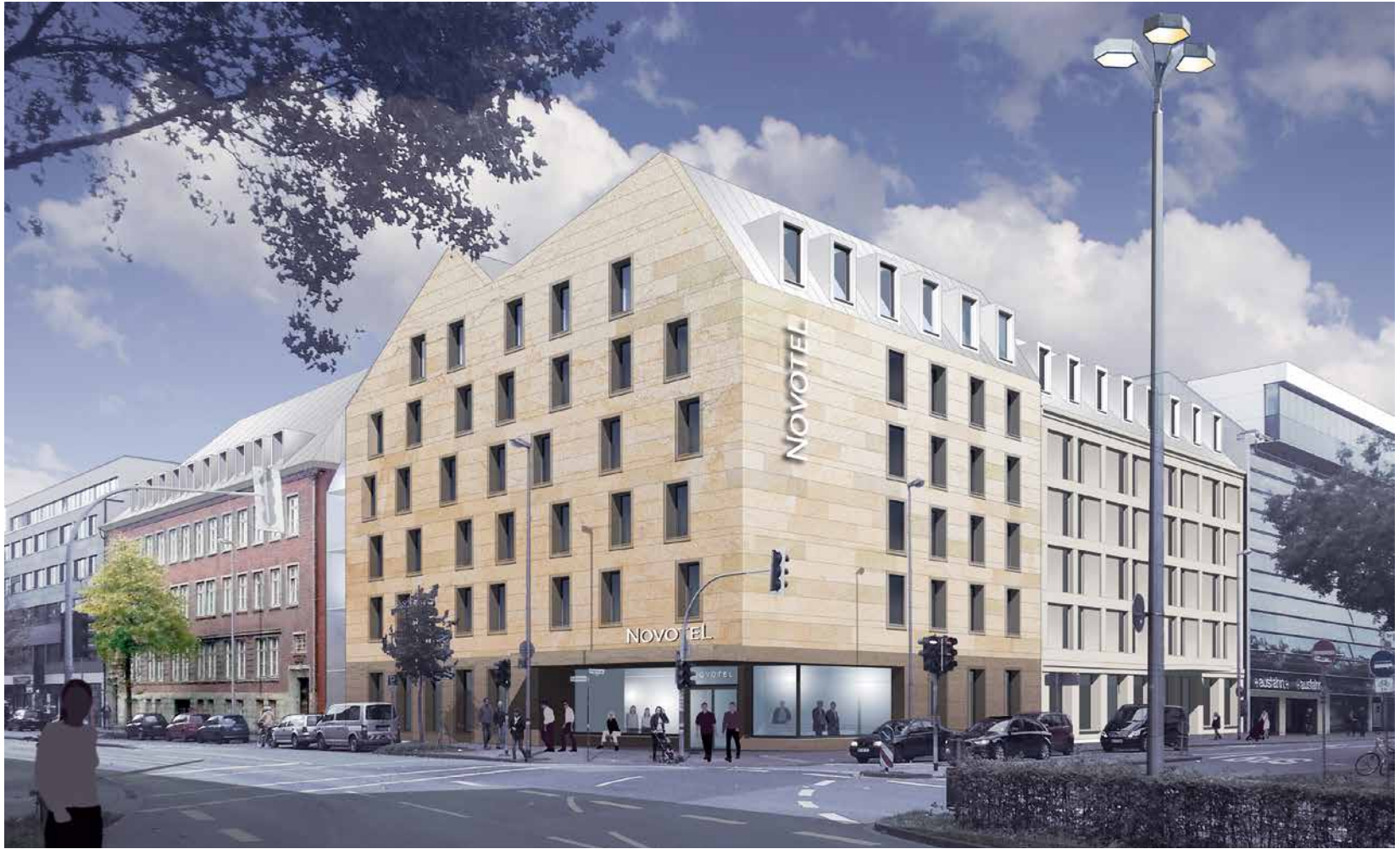
The two new buildings on the corner. Architecture and draft: PSP Weltner Louvieux Architekten
