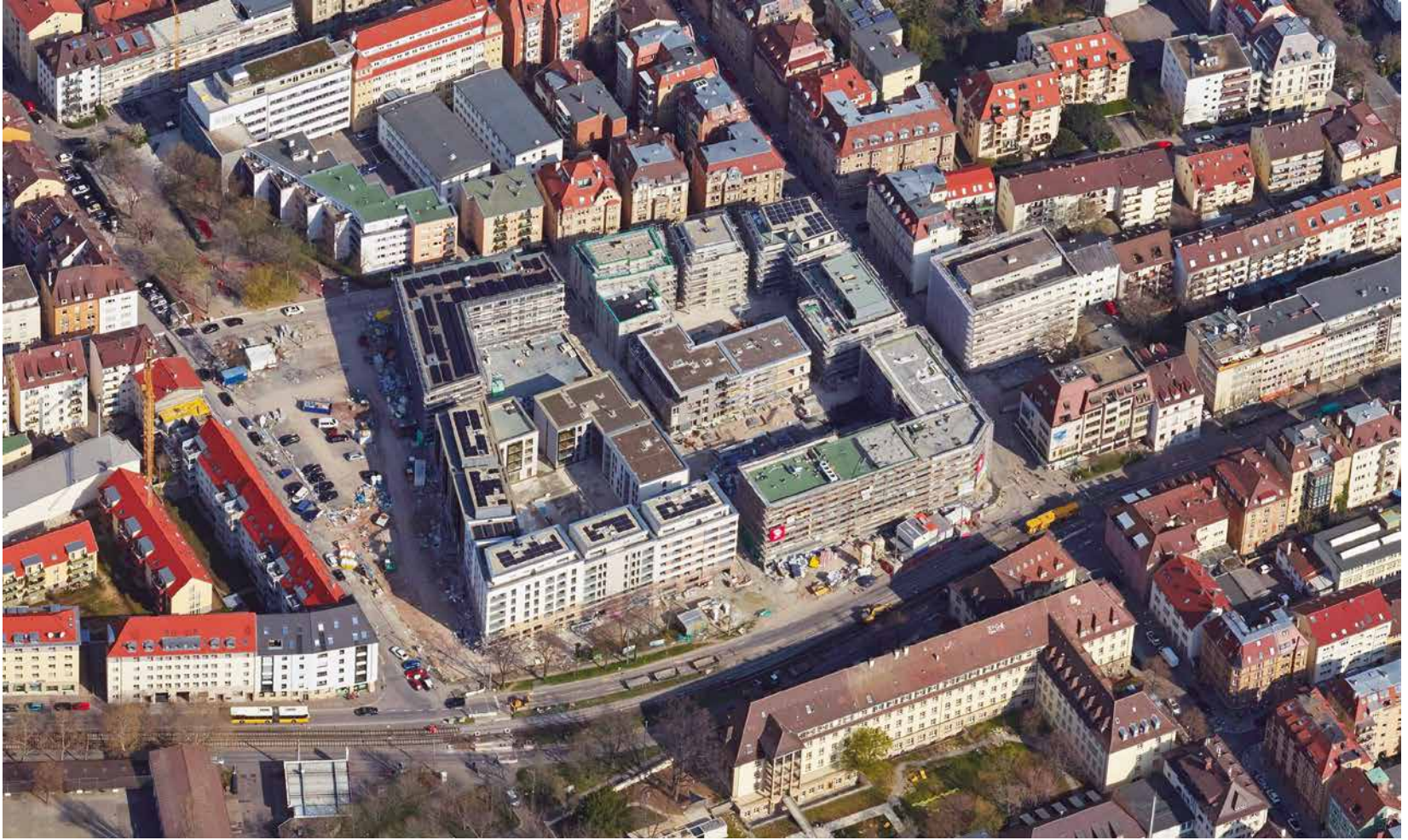
Aerial photo of the finished Olga Plot. Photo: Landeshauptstadt Stuttgart
