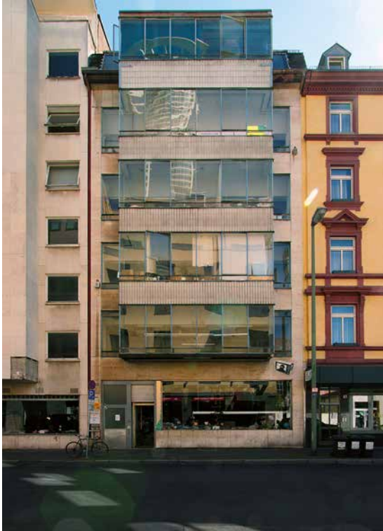
The building at Niddastraße 59 prior to remodelling. Photo: Ulrich Becker
