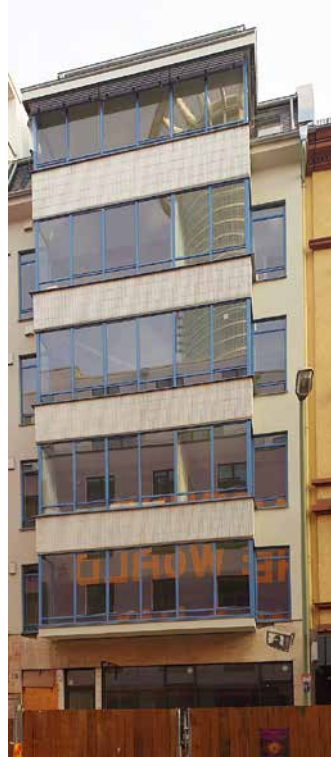
The old Niddastern building, with its new steel-framed windows. Photo: RT
