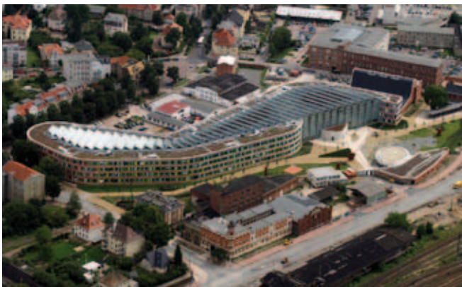
Umweltbundesamt Dessau (Federal Environment Agency Dessau): Urban Space Situation (Photo: Busse)
