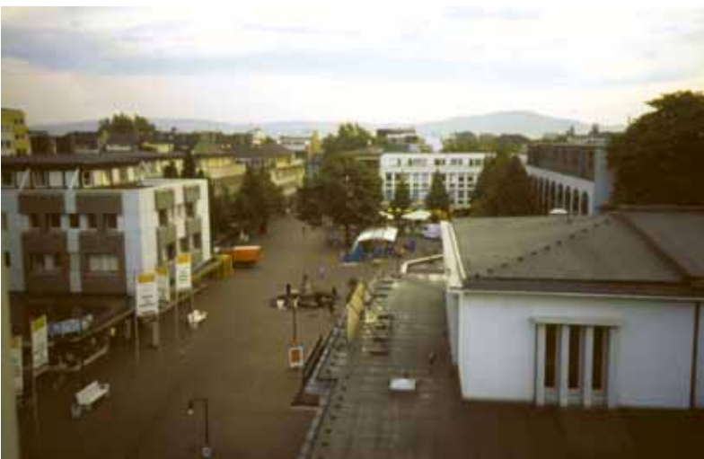
Bonn-Bad Godesberg: Extensive Replacement New Construction and Pedestrian Precinct
