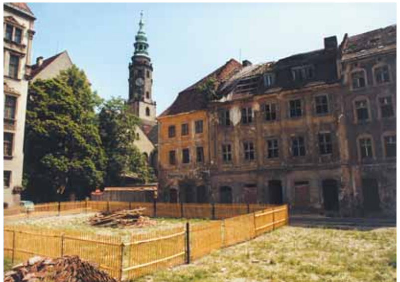
Görlitz: Building Damage in the Old Building Stock
