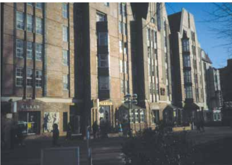
Rostock Old Town: New Replacement by Pre-Fabricated Buildings with Special Elements
