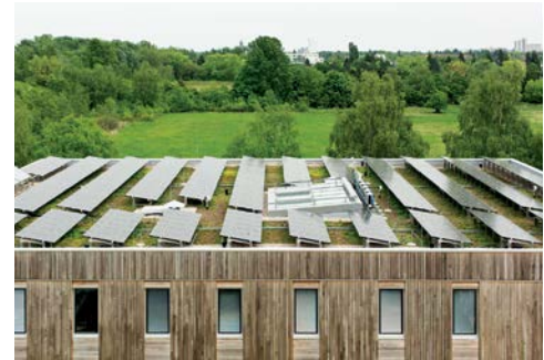
Left: South elevation of the building Right: View of the roof with photovoltaic modules and solar thermal collector
