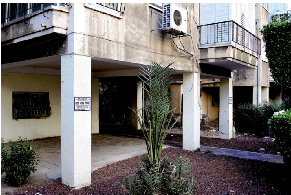
Figure 41: Here, a ground floor entrance that is open to the street translates into an optically wider street and provides shade for the building entrance (Tel Aviv, 2013)
