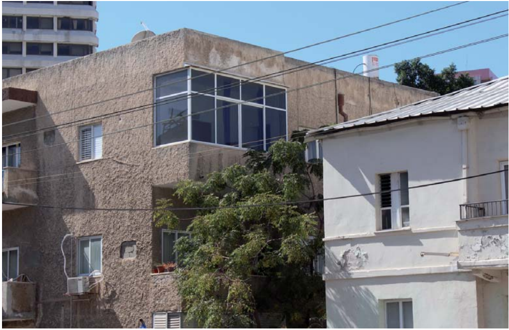
Figure 65: Plasterwork, Idelson Street, Tel Aviv (2013)
