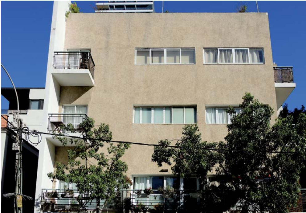
Figure 46: Cantilevered facade slabs (left) capture the ocean breeze (Tel Aviv, 2013)
