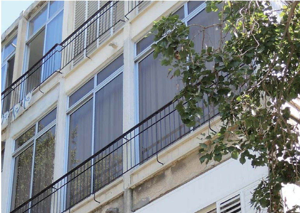
Figure 49: Glassed-in balcony with interior shading elements (Tel Aviv, 2013)
