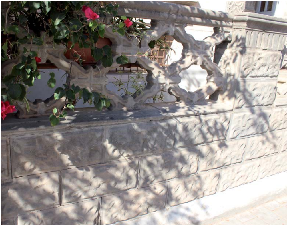
Figure 108: Characteristic street-side garden walls made of precast concrete blocks; Neve Tsedek, Pines Street 30, Tel Aviv (2013)
