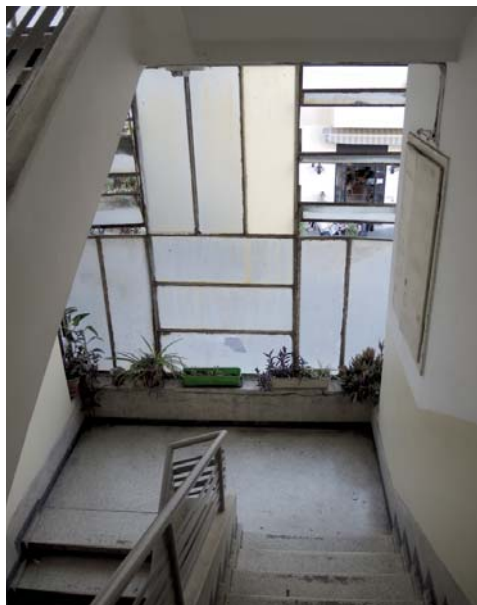
Figure 83: Interior view of staircase at Pinsker Street 23 in Tel Aviv (2013)
