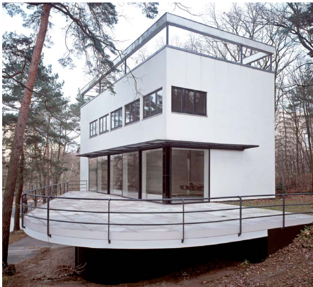
Figure 26: Oblique (southwest) view of the building at Am Rupenhorn 25 in Berlin (photo: Christian Gahl).
