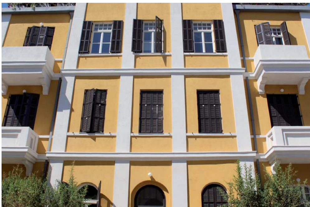
Figure 102: Eclectic-style apartment building with two added floors; Ahad Ha'am Street, Tel Aviv (2013). The entire third floor and the recessed penthouse were added in 2013. The only visible traces of this change are the reduced forms of the balcony balustrades.
