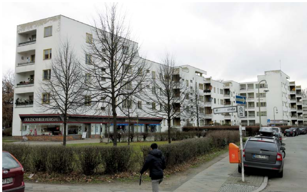
Figure 25: Großsiedlung Siemensstadt "Panzerkreuzer," Berlin-Charlottenburg, southeast view (2014)
