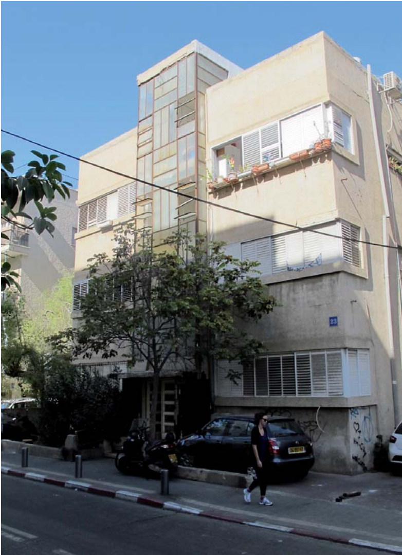
Figure 82: Elaborate steel frame windows, in a checkerboard pattern, in a staircase at Pinsker Street 23 in Tel Aviv (2013)
