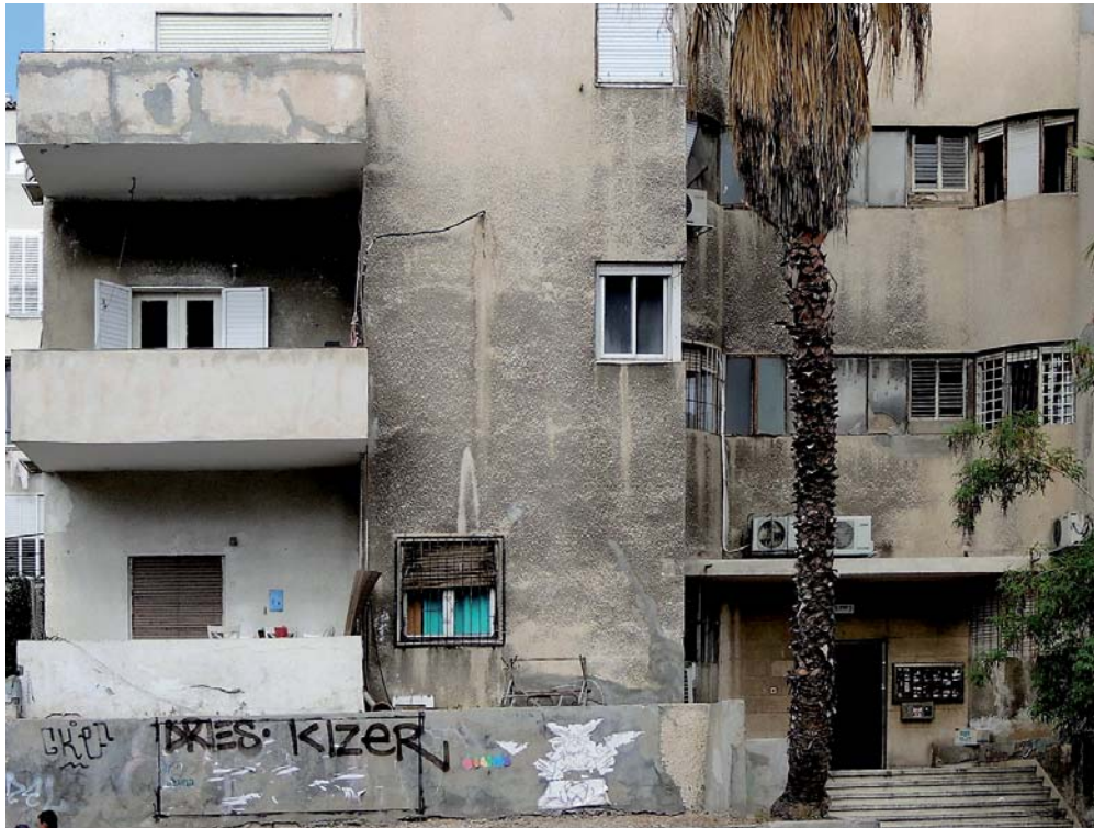
Figure 52: Facade soot particles (Tel Aviv, 2013)
