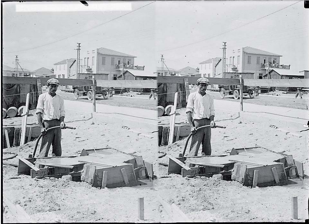
Figure 109: Foundation concreting at a Tel Aviv construction site (stereo photograph, around 1930).
