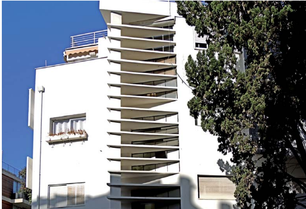
Figure 53: Clean, white facade (Tel Aviv 2013)
