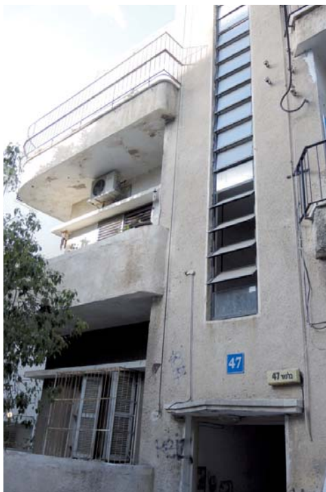
Figure 76: "Thermometer" windows with steel frames and movable panels; Tel Aviv (2013)
