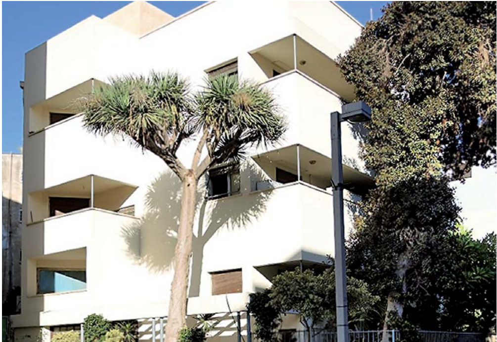
Figure 40: Light coloured plaster facade with small windows, most of which are recessed and are thus shaded by the balconies; Idelson Street 29, Tel Aviv (2013)
