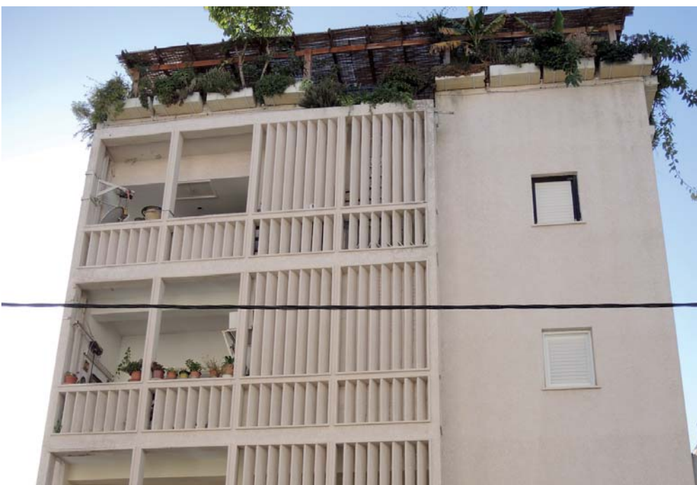
Figure 47: Vertical slats capture the ocean breeze and provide shade (Tel Aviv, 2013)
