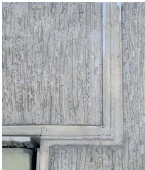
Figure 73: Decorated facade plasterwork (Tel Aviv 2013)
