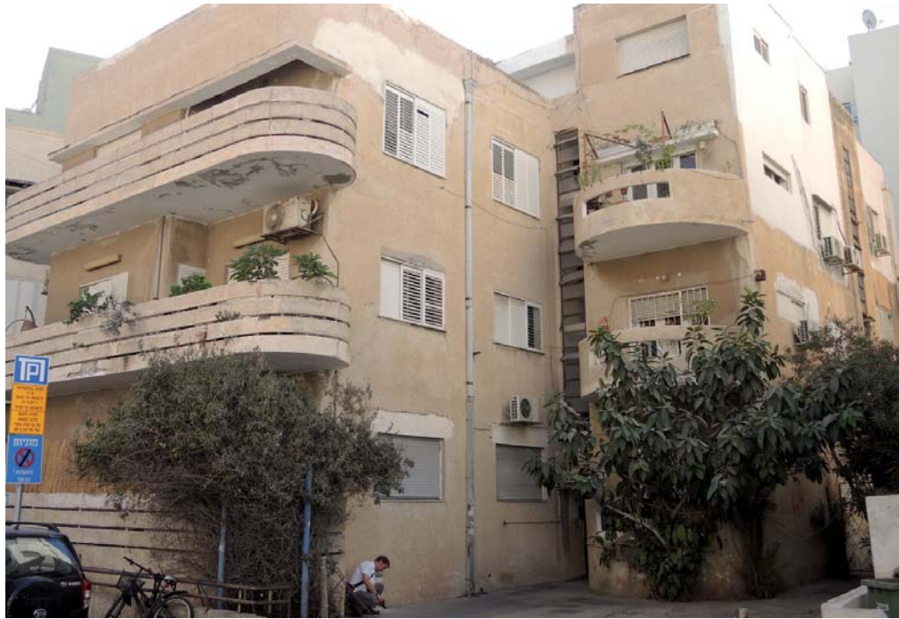
Figure 44: Vertical ribbon windows that allow for staircase ventilation; Idelson Street 14 (Tel Aviv, 2013)
