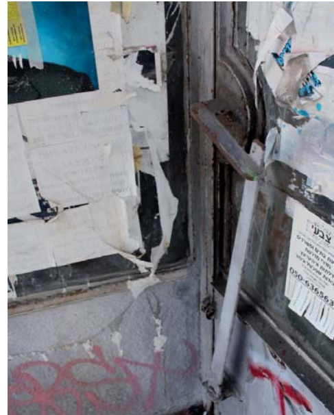
Figure 84: Fully preserved steel frame glass door (store entrance), Allenby Street 52, Tel Aviv (2013)
