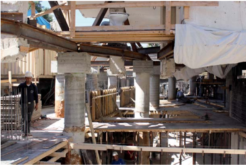
Figure 96: Large construction site, Hen Street, Tel Aviv (2013)
