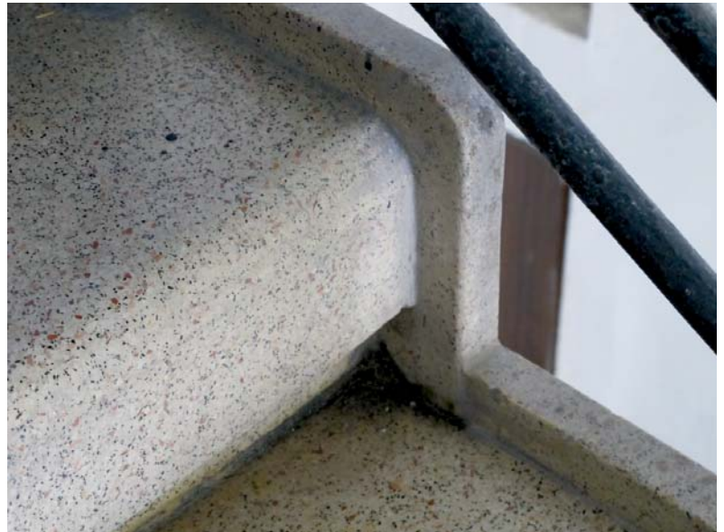
Figure 80: Staircase with terrazzo cast steps and added coloured stone aggregates; Aharonovitch Street 30, Tel Aviv (2013)
