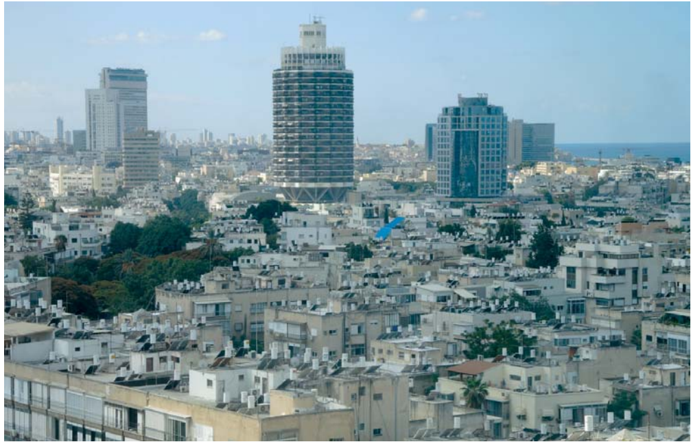
Figure 56: Thermo-siphon installations on rooftops in downtown Tel Aviv (2013)
