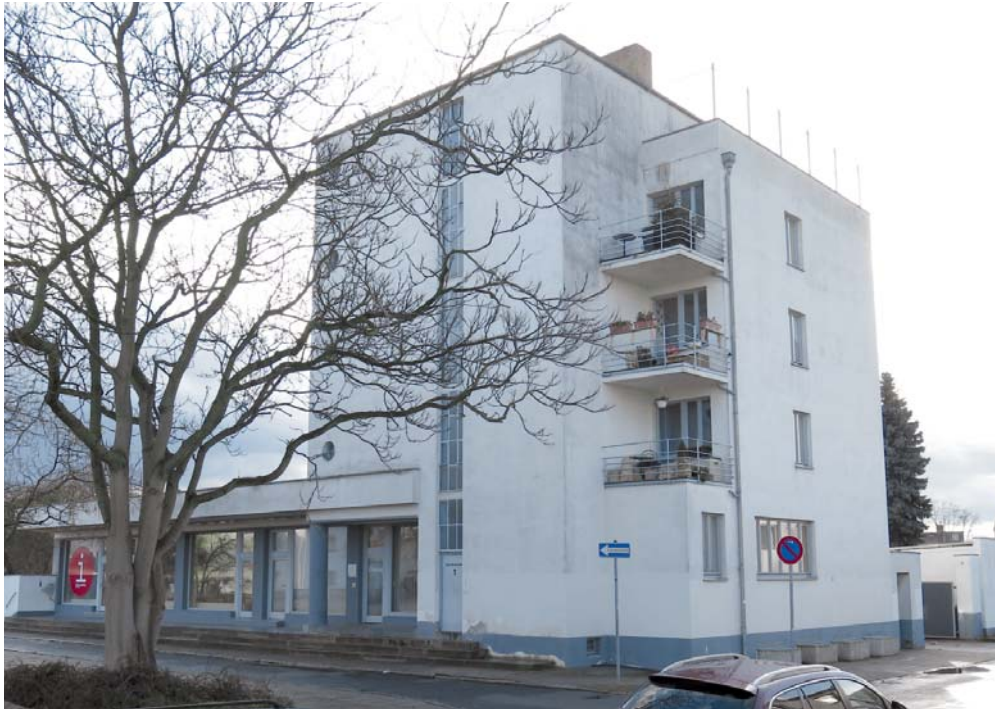
Figure 24: Konsumverein building, Dessau-Törten; northwest view (2014)
