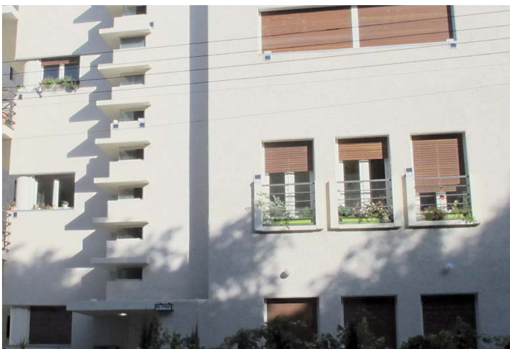
Figure 43: Shade created by cantilevered cement slabs (left) and roller blinds (right) (Tel Aviv, 2013)
