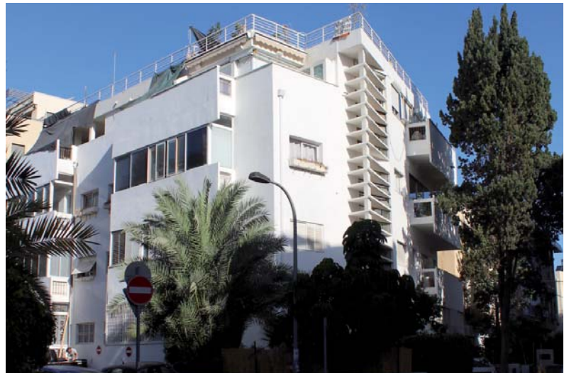
Figure 101: Corner apartment house with an added floor, Frug Street, Tel Aviv (2013)
