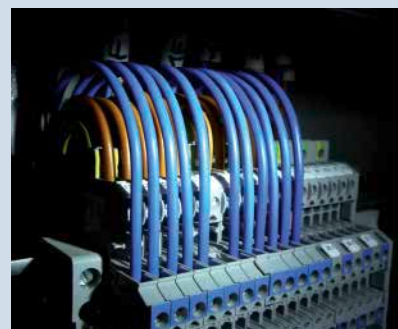
Figure 95: Measurement server Photograph: Fraunhofer IBP
