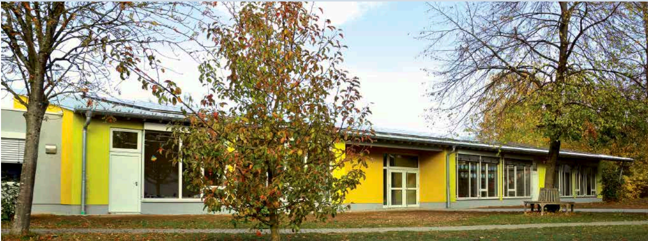
Figure 63: View of the extension's south side Photograph: Haase & Bey Architekten
