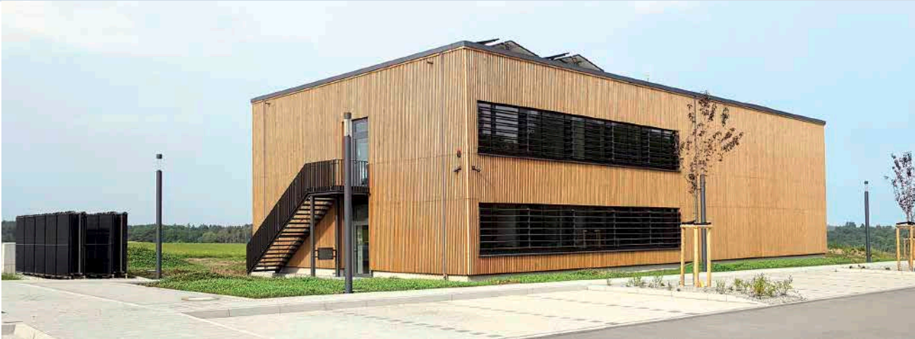
Figure 51: View from the south-west towards the research hall and the adjacent solar air absorber block Photograph: Dr Reinhardt Reck
