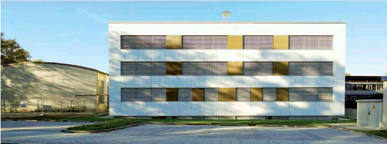
Figure 28: View from the south towards construction segment 1 Photograph: ARIS Architekten
