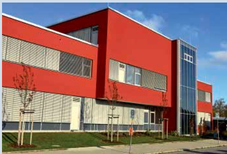
Figure 19: Partial view of the building's south side Photograph: Winkler-Architekten
