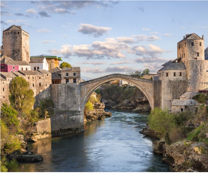
Fig. 23: Stari Most bridge. Mostar, Bosnia and Herzegovina (iStock.com/Ozbalci)
