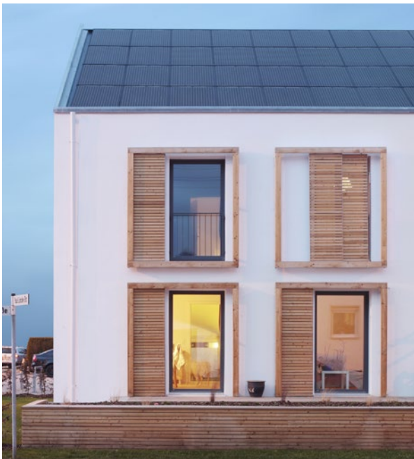
Efficiency House Plus, Pfuhler Strasse 12-14, Neu-Ulm, with photovoltaics integrated into the roof
