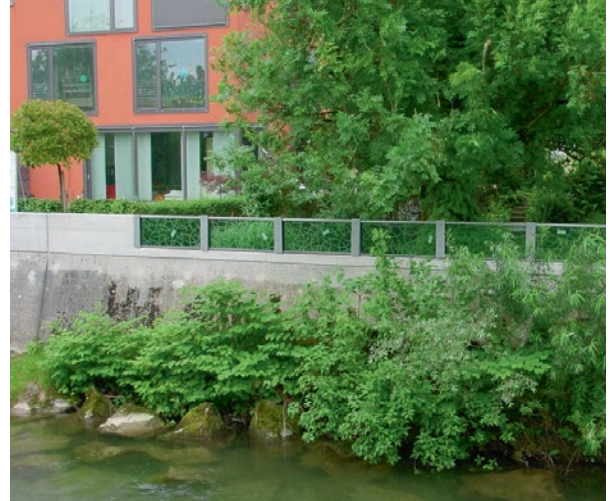
Flood protection wall made of safety glass
