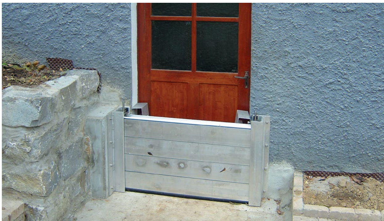
Flood protection for building openings
