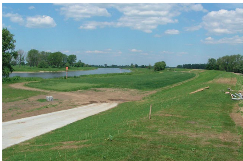
Flood protection dike along the Elbe River
