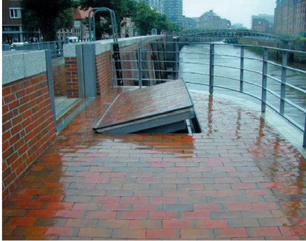
Integrated flap gate for flood protection
