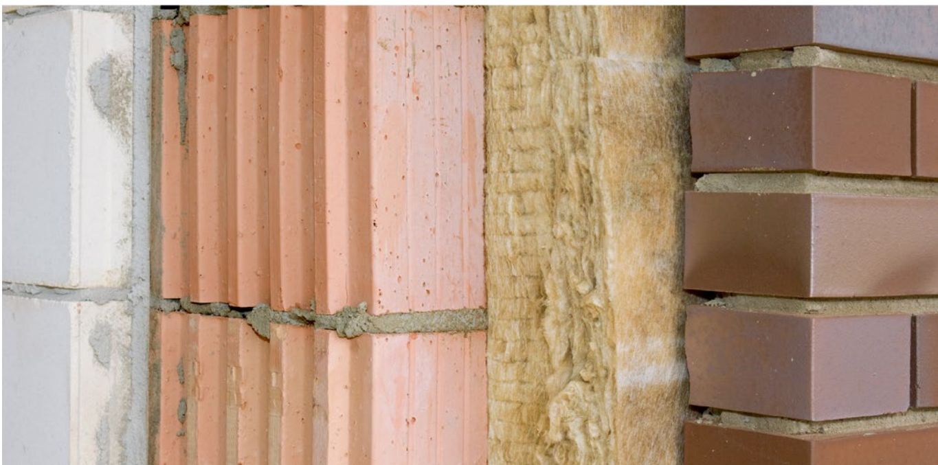
Multi-shell exterior-wall structure
