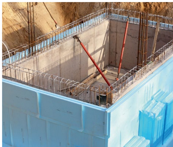
Waterproofed cellar with thermal-insulation layer
