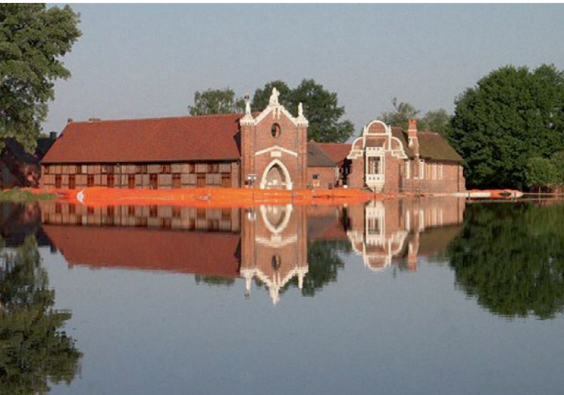
Flood protection with mobile, water-filled tube system
