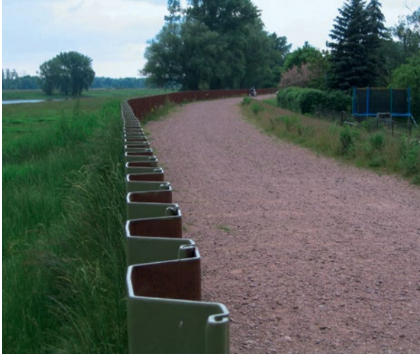
Flood protection wall built with steel sheet piles
