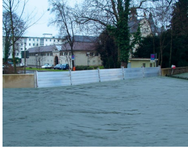
Mobile flood protection with bulkheads
