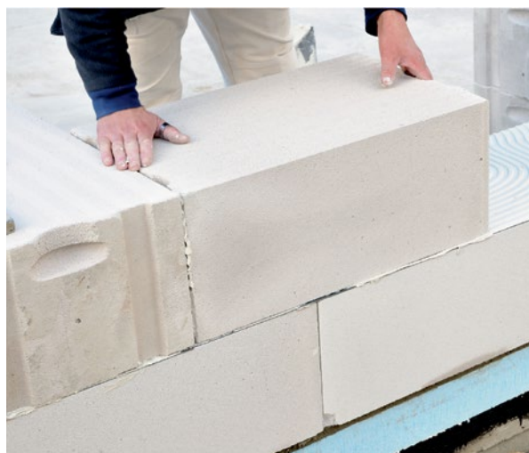
Wall built of aerated-concrete blocks
