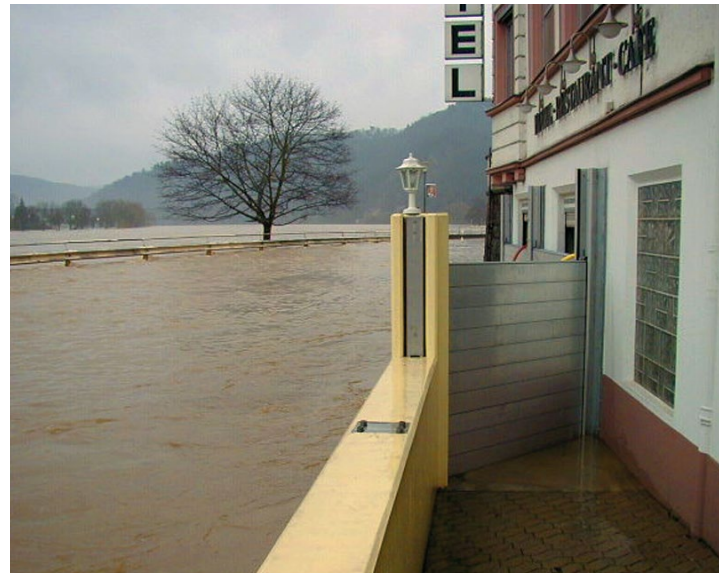
Circumferential flood protection with partly mobile wall elements
