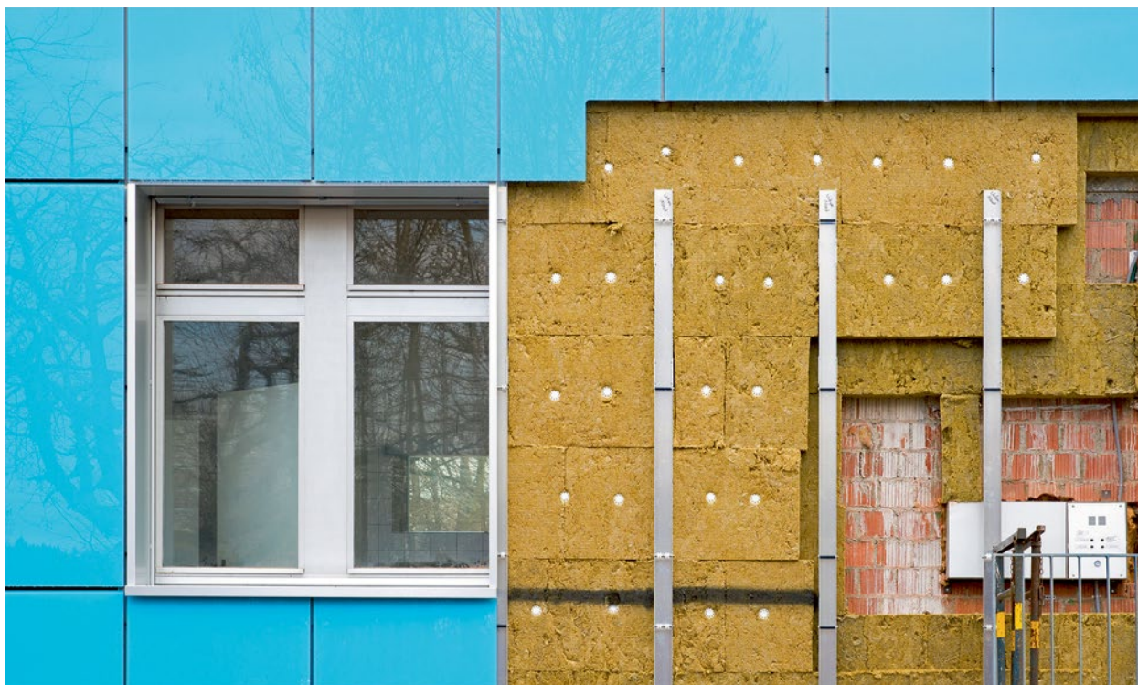
Back-ventilated facade construction
