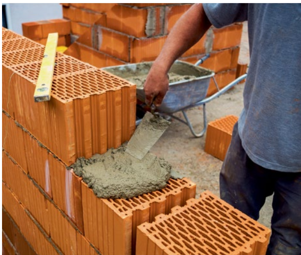
Wall of vertically perforated bricks with low bulk density
