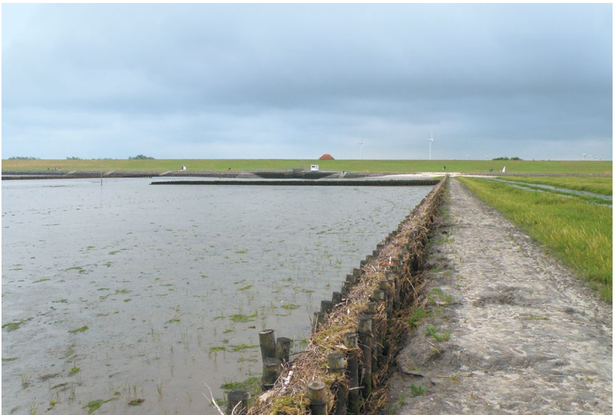
Coastal protection with groynes and a flood control dike
