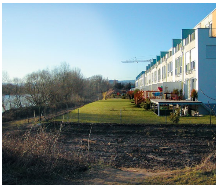
Flood-adapted construction, with raised ground floor
