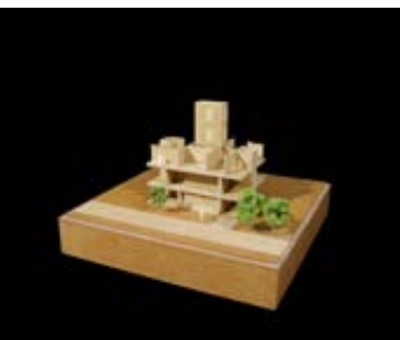
... and the prefabricated wooden storeys are hung on the stairwell core.
